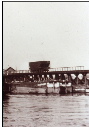
Railroad coal car on the trestle above the canalboats. A door in the bottom of the car allowed coal to drop by gravity into the boats.
