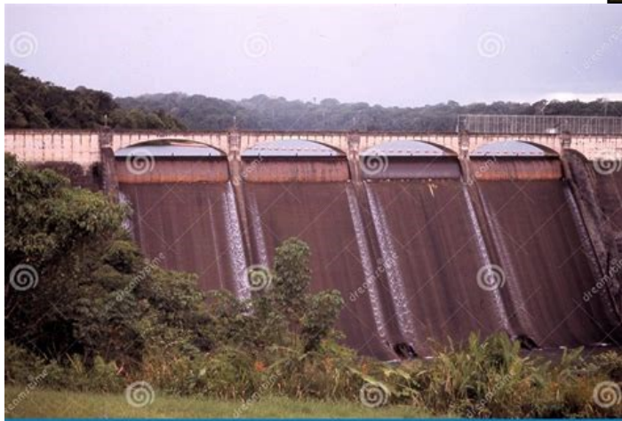
This very large spillway takes excess water from Gatun Lake, a part of the Panama Canal. During the rainy season, the lake can easily overflow.
