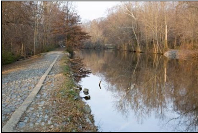
A typical spillway (on left) along the D&R Canal. This spillway is part of the towpath and is made of stone to prevent the erosion of the towpath.
