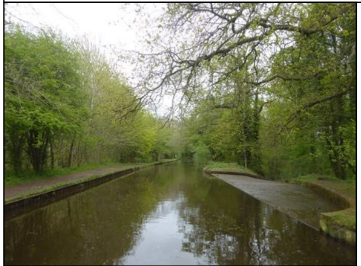
This spillway (on the right) controls the level of the Llangollen Canal in Wales.
