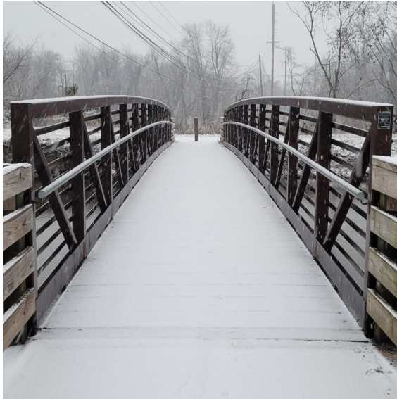
Pedestrian bridge at Demott Lane Photo by Shaun Daley
